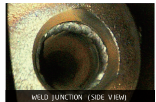
WELD JUNCTION (SIDE VIEW)
