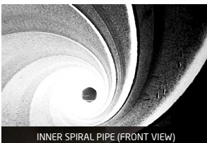
INNER SPIRAL PIPE (FRONT VIEW)
